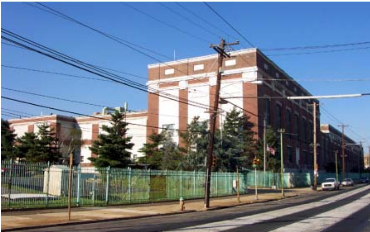
The General Electric site at 6739 Elmwood Avenue, where 7,000 individuals were once employed, is one of Southwest's largest and most significant redevelopment sites, located in the heart of the Elmwood neighborhood. It is anticipated that the site will need extensive environmental remediation.
