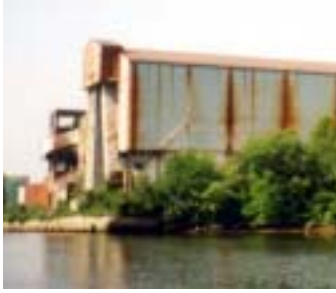
Land assembly on the Schuylkill waterfront, including a waste/recycling area (above) and the US Gypsum site (below), is a first step towards redevelopment.
